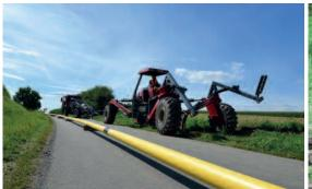
Surface after installing a drinking water pipeline 250 x 14.8 with the Rocket Plow.
