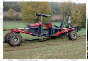
Plowing in of a sewer pressure pipe HDPE OD 90.
