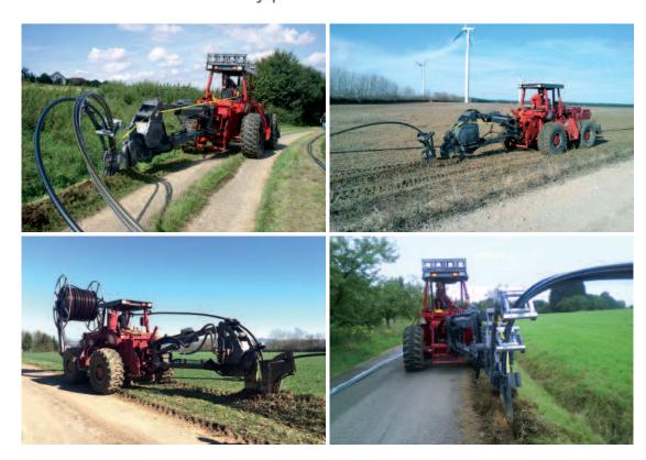
Plowing in of a cable protection pipe HDPE OD 50.
